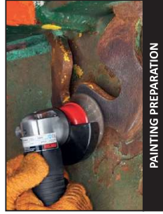
WELD SEAM REMOVAL
